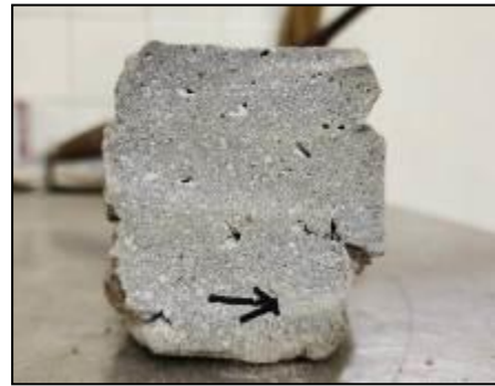
Fig -31: Core Samples cross section examination. No serious cold joints, shrinkage cracks or voids found
