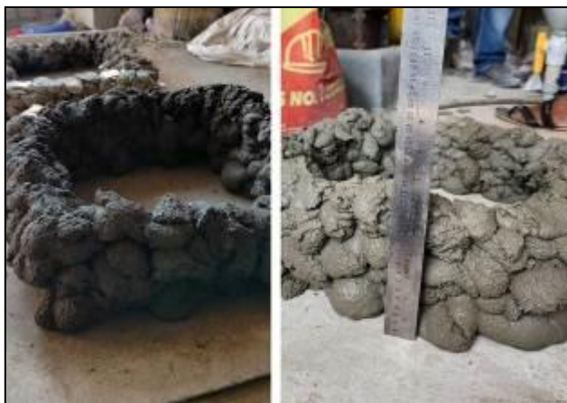
Fig -43: Left - Extrusion completed & Right – Improved Buildability with respect to Trialmix-01
