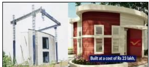
Fig -4: COBOD gantry type printer (BOD 2) & India’s first 3D printed post office building at Bangalore made with COBOD printer, constructed by L & T. 1000sqft in 45 days, Crew of only 5 peoples. Cost 23 lakhs. Life span 50 to 100 years
