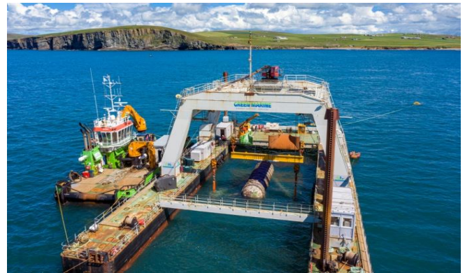
Fig 2 - Microsoft under water data centre
