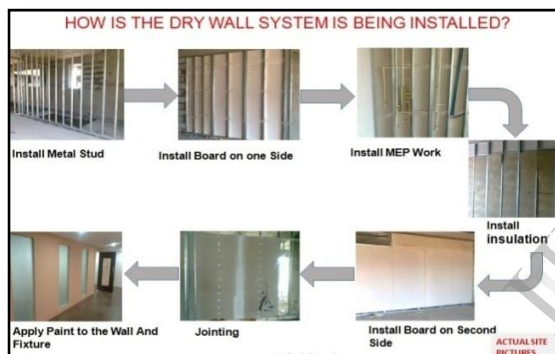
Figure 2: installation procedure of Dry Wall
