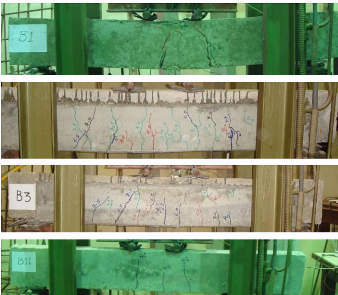
Fig. 10. Crack pattern for control, strengthened and retrofitted beams
