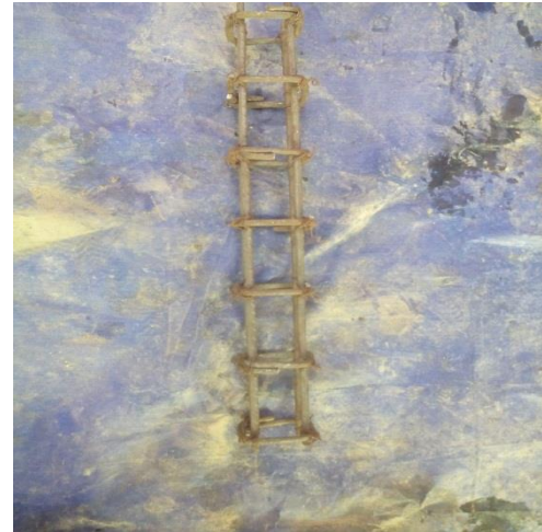
Fig 5:-Reinforcement of 6mm dia
