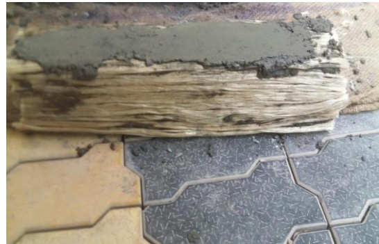
Fig 10:-Retrofitting on three sides of beam
