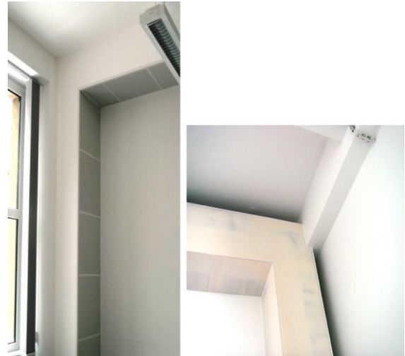
Figure 1. Application of mineral wool absorber behind plaster board covers [11]
