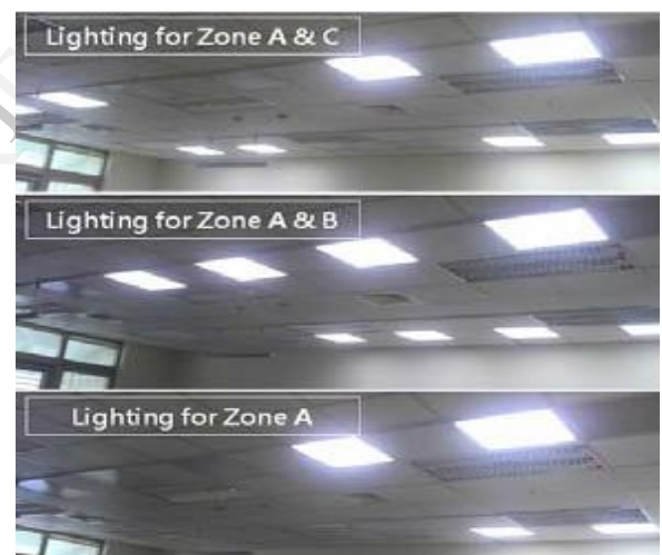
Fig. 6 Controls for dedicated lighting zone
