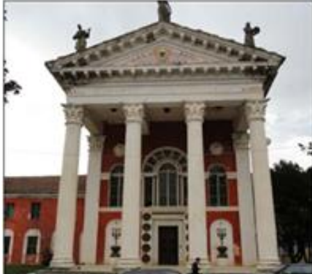
Figure 3.1 Frontal view of the building
