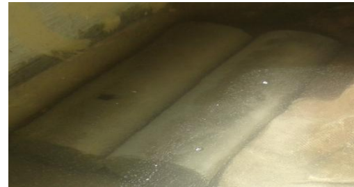
Fig 3 : Curing of column
