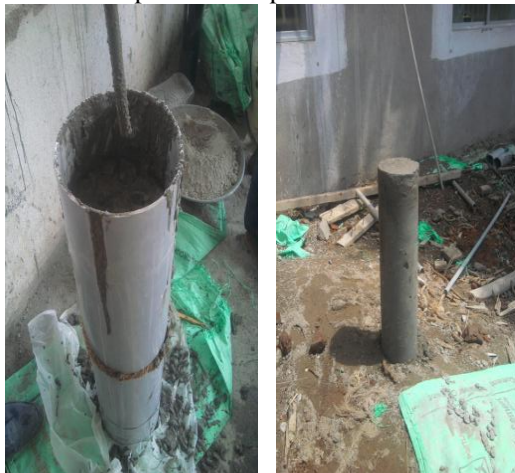
Fig 2 : casting of column
