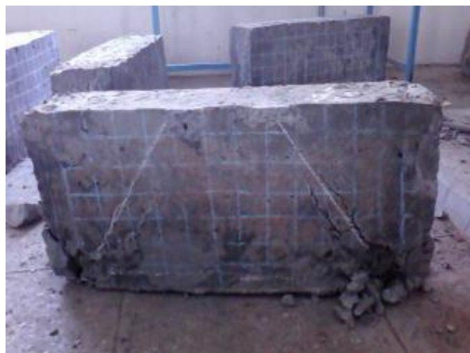
Image 9 Strut formation in deep beams
