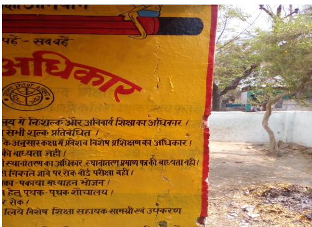
Figure 4:- Corner Wall Crack
