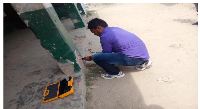
Figure 1 :- Rebound Hammer Testing
