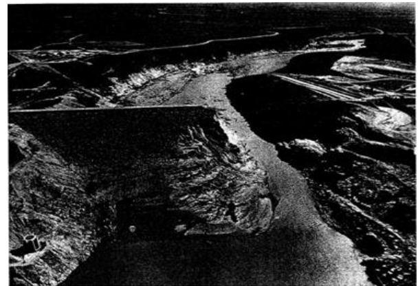
Figure 1: View of failed Teton dam
