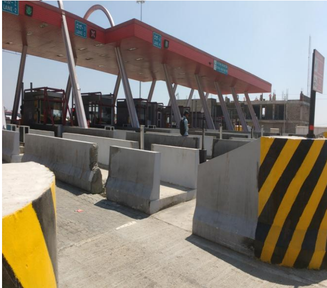
Figure 1.1: Toll plaza of the Study Area.
