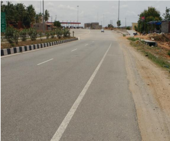
Figure 3.1: Showing the Flexible Pavement and rigid pavement near the Toll Plaza.
