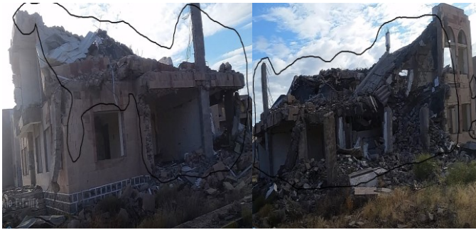
Fig. 12. General view of damaged building in Jahana
