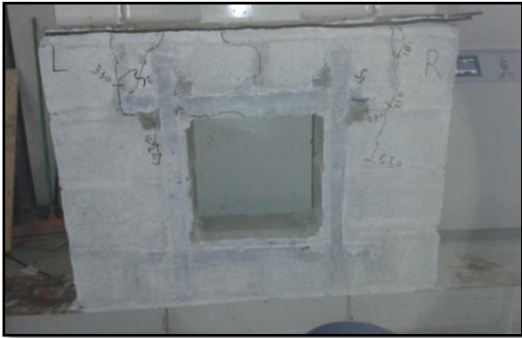
Figure (15) Failure modes of specimen WC2
