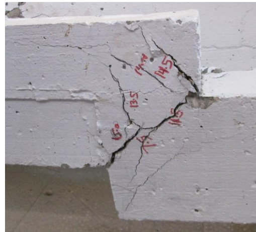
Fig. 3. Crack pattern of experimental tested beam
