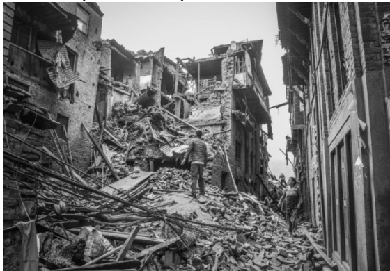
Fig1: Failure of soft storey building due to earthquake.
