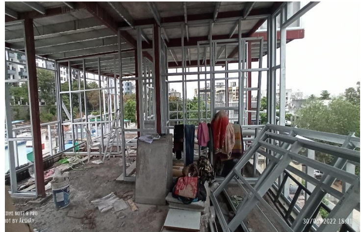
Fig. 4. Erection of LGS Frames
