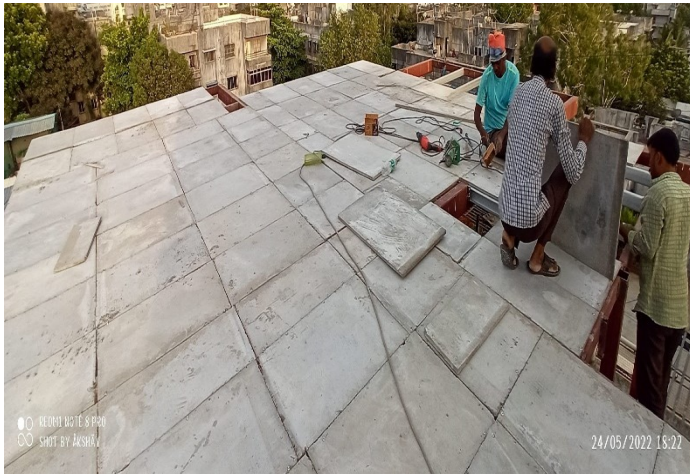
Fig. 3. Fixing of Ferron panels
