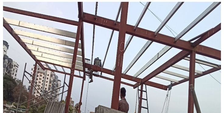
Fig. 2. Fixing of Joist member for Slab
