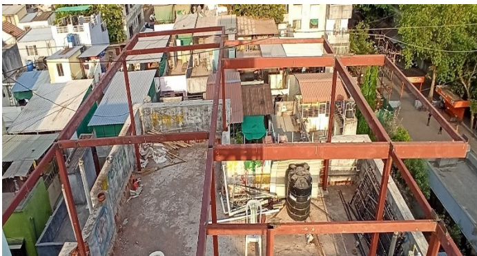
Fig. 1. Erection of MS Columns, Beams
