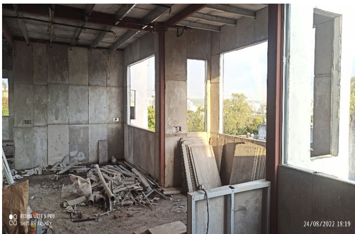
Fig. 5. Fixing of Ferron panels for walls
