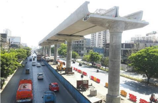
fig: Mumbai Metro U girder
