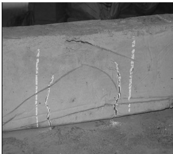
Fig7. Crack pattern in beam reinforced with Proposed rebar.
