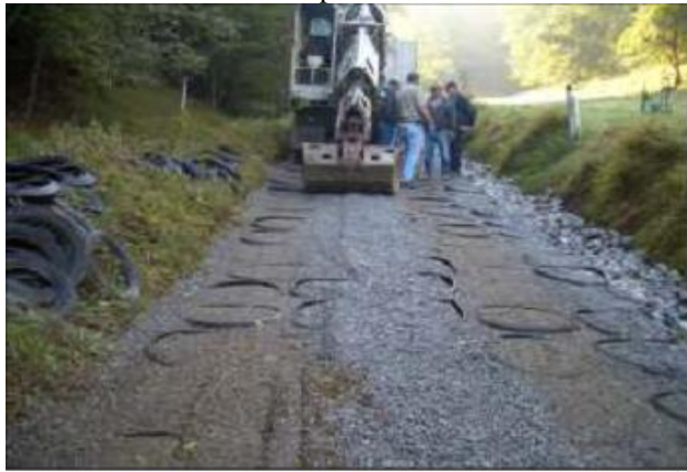
Fig.6. CA Concrete base
