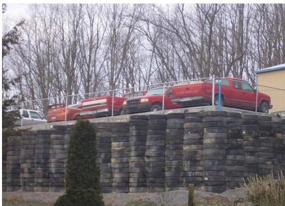
Fig.8. Confined Aggregate Concrete as a Retaining wall
