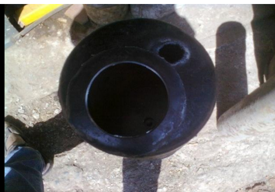
Figure 2.4-Cutting flange for tank
