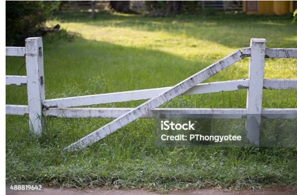
Figure 3: Villagers' broken fence, damaged by animals, left unrepaired for years.
