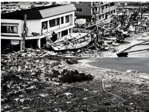
Fig 1. Japan earthquake and tsunami of March 11, 2011.
