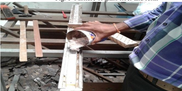
Fig. 2 Pouring of glass fiber and resin mixture
