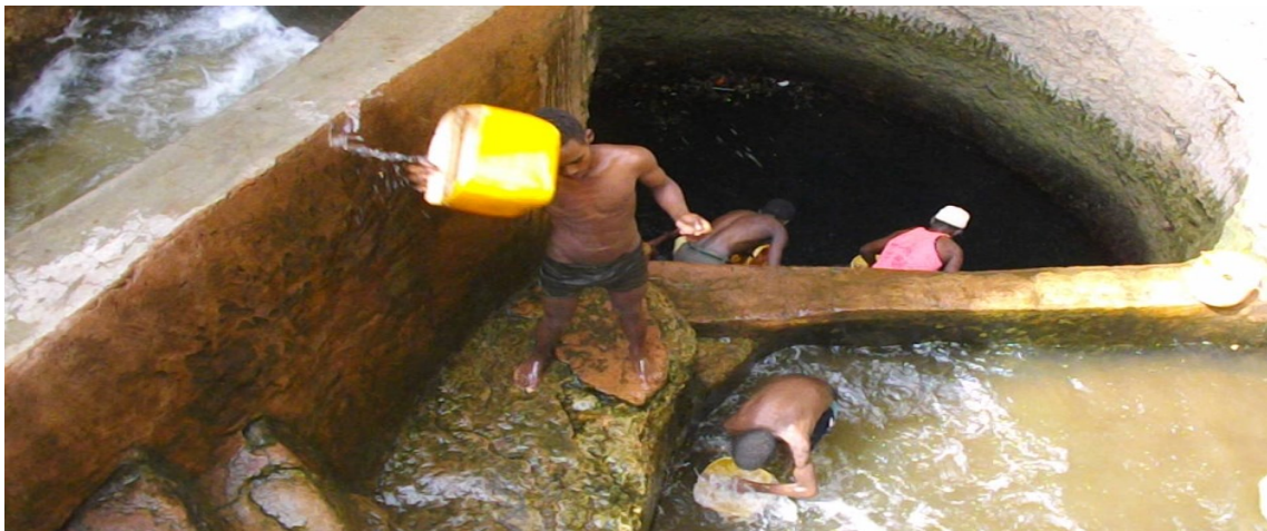
Figure 5 Madda or qaa'a eelaa (the borhole), Faccana and Koloco structures of Tula well at Gorile (eela Odicha), showing that how water lose by traditional lifting method.
