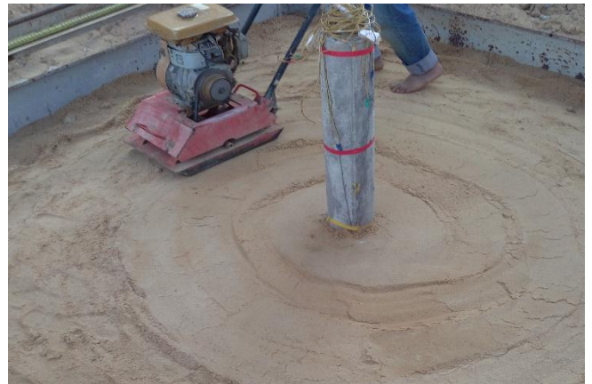
Fig. [10] Placing Soil around Tested Pile for group (1) - Single Pile
