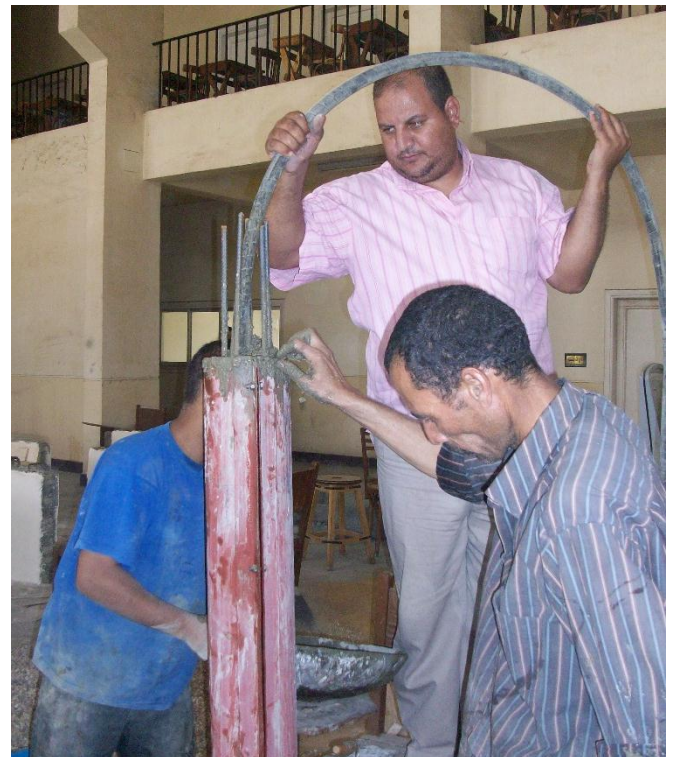
Fig. [5] Casting of Piles
