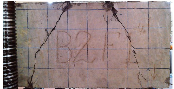
Fig 19 Crack Pattern of beam D40 AR50 [F1%]
