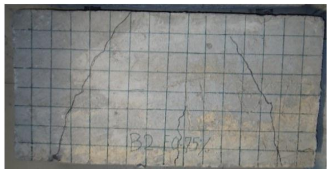
Fig 8 Crack Pattern of beam D40 AR80 [F0.75%]
