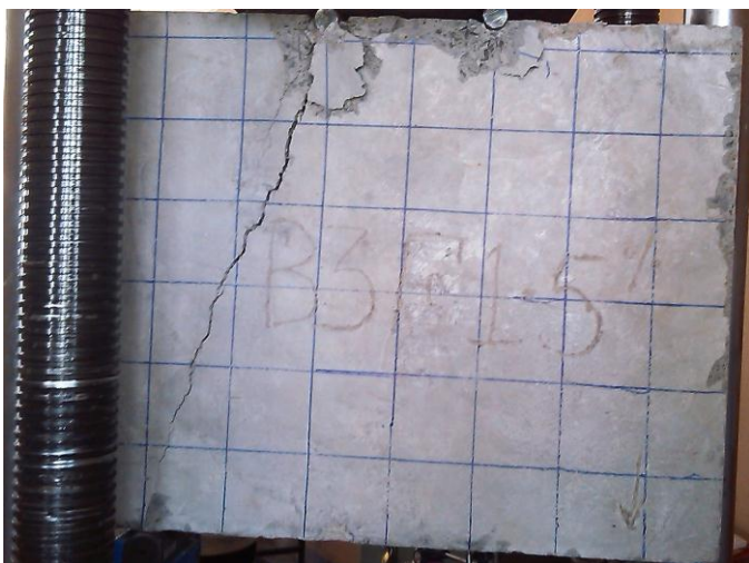
Fig 24 Crack Pattern of beam D60 AR50 [F1.5%]
