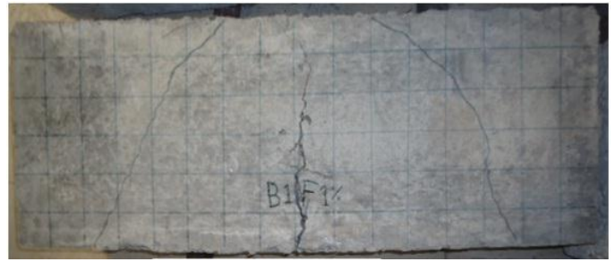
Fig 5 Crack Pattern of beam D30 AR80 [F1%]
