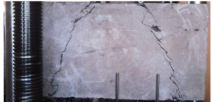
Fig 20 Crack Pattern of beam D40 AR50 [F1.5%]
