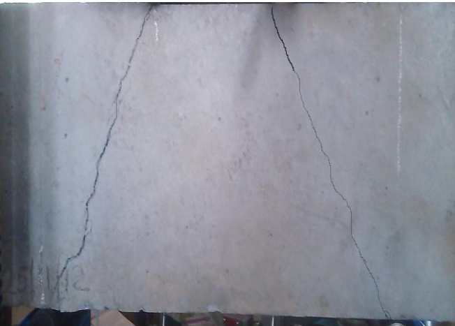
Fig 10 Crack Pattern of beam D60 NRC [F0%]
