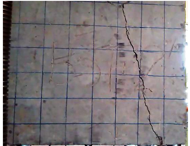
Fig 25 Crack Pattern of beam D60 AR50 [F2%]
