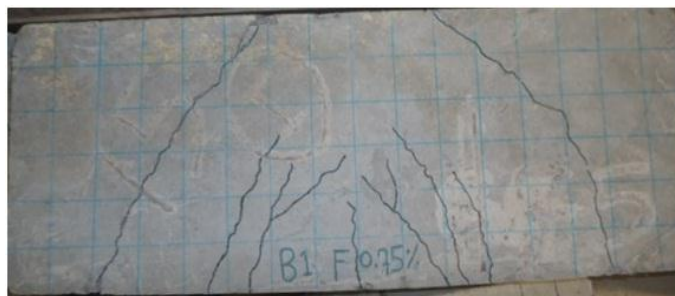
Fig 4 Crack Pattern of beam D30 AR80 [F0.75%]
