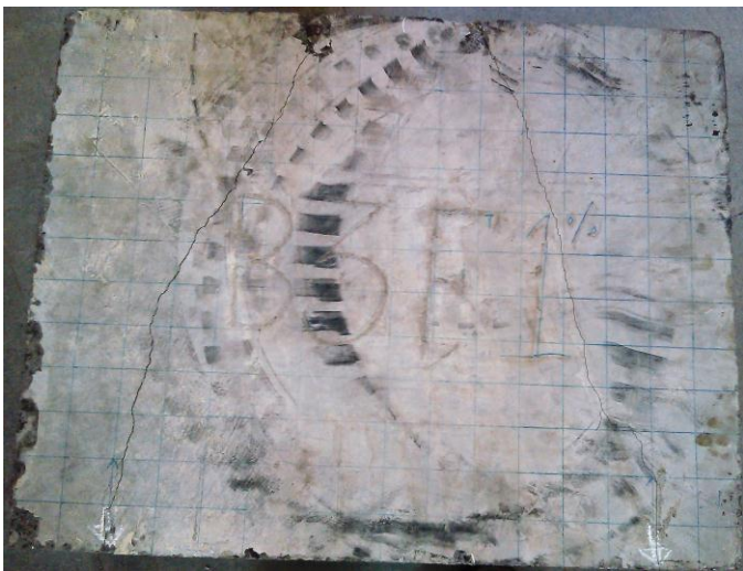
Fig 23 Crack Pattern of beam D60 AR50 [F1%]
