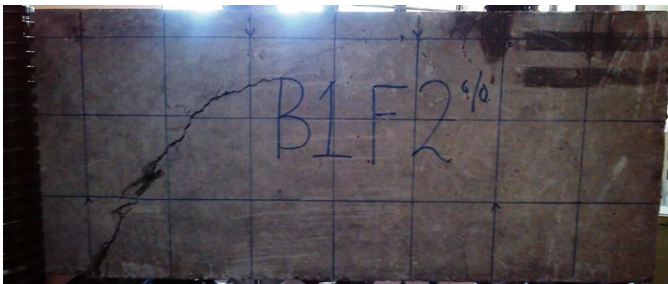
Fig 17 Crack Pattern of beam D30 AR50 [F2%]
