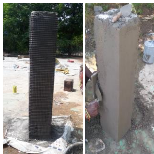
Fig. 1 Retrofitted column
