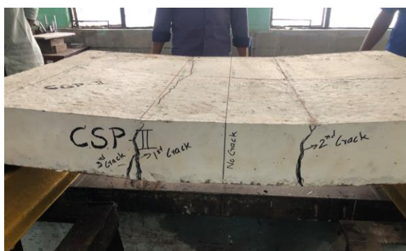
Fig. 6: Flexural Cracks formation of CSP - II
