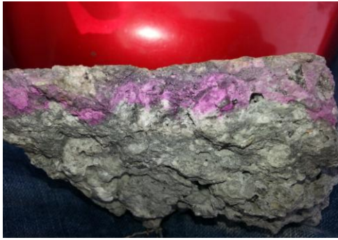
Fig 5: Depth of carbonation.
