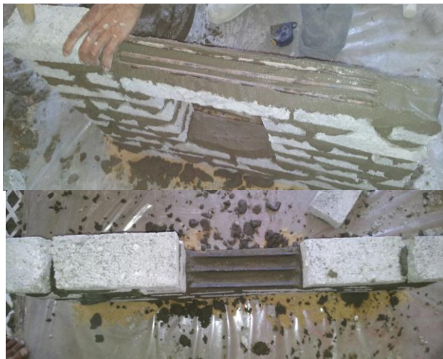
Fig. 8. Strengthening brick walls with opening using 3Ø8 steel bars embedded into bed joint mortar above lintel and sill with length (L2 = 65 cm)
