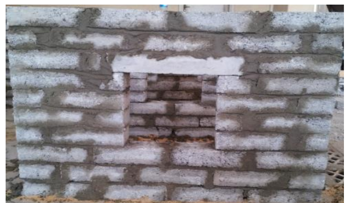
Fig. 3. Brick wall with R.C.lintel 35 cm (control wall)
