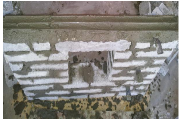
Fig. 6. Strengthening brick walls with opening using 3Ø8 steel bars embedded into bed joint mortar above lintel only with length (L3 = 85 cm)
