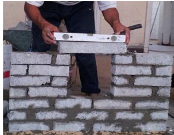
Fig. 2. Brick wall specimen during construction
