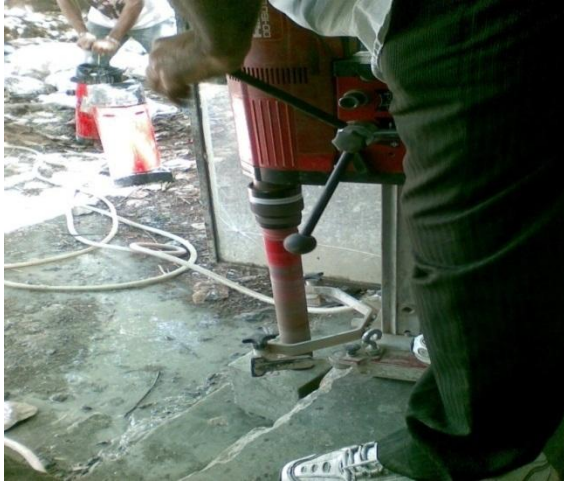
Figure 1. Core drilling machine
