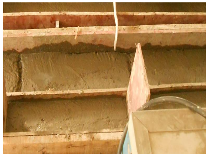
Figure 5 (Retrofitting of beams)
