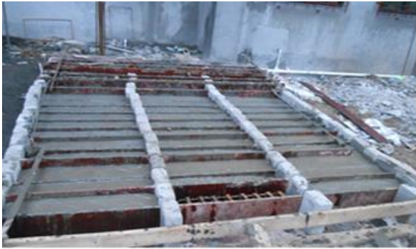
Figure 3 (Casting of beam.)
