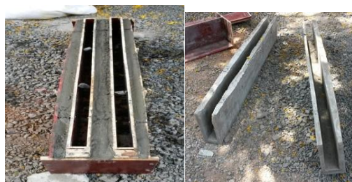
Fig 4.2 Casting and form of U-shaped Ferrocement beam
