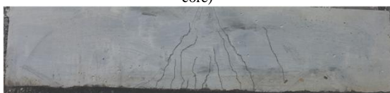
Fig 11.2 Beam - Hsb2 (Single layered Hexagonal wire mesh with brick core)
