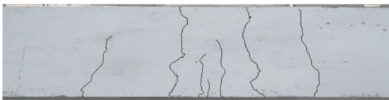
Fig 7.1 Beam - Wdc1 (Double layered welded wire mesh with concrete core)
