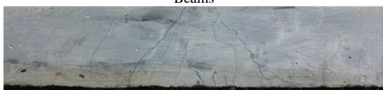
Fig 11.1 Beam - Hsb1 (Single layered Hexagonal wire mesh with brick core)
