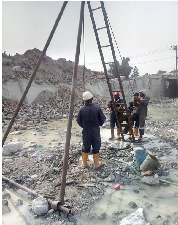
Fig. 3: Field crew drilling at the collapsed building site.
