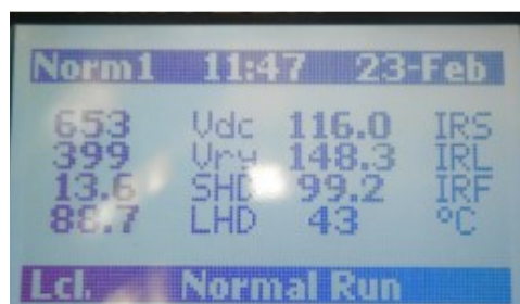
Fig 7.7 b Source Harmonic distortion -13.6 % at 50 % AHF rating ( 99.2 A)
