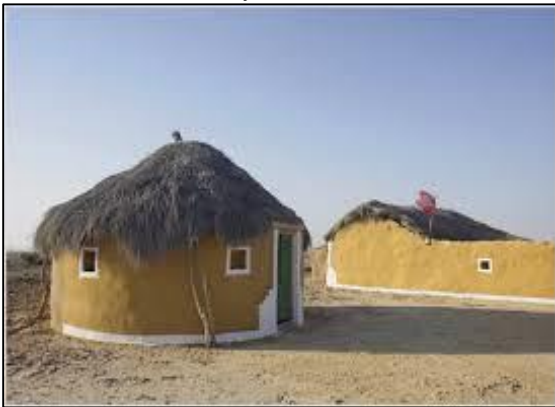
Fig. 2. Small opening used as a Window in Northern Rajasthan [19]
