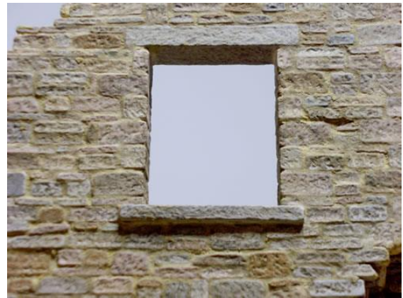
Fig. 13. Stone patti Lintel instead of R.C.C. Lintel[19]
