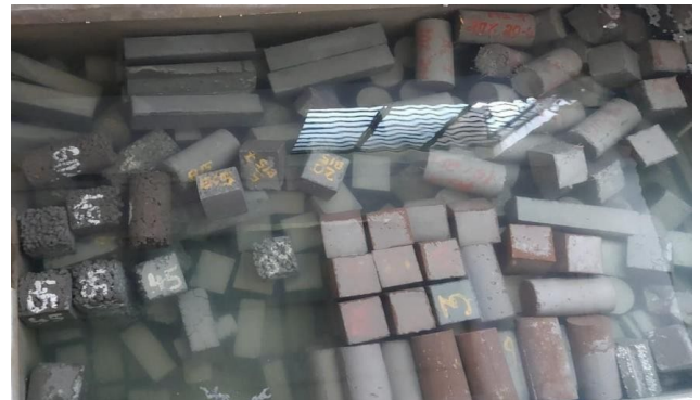
Fig 4 Curing of Concrete (Moulds)
