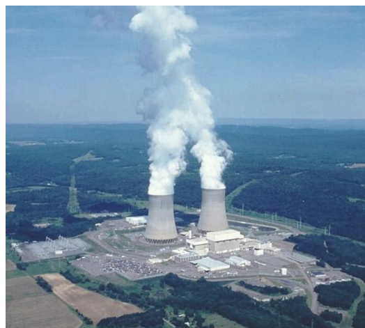
Figure 4 -The Susquehanna Steam Electric Station, in Pennsylvania, United States
