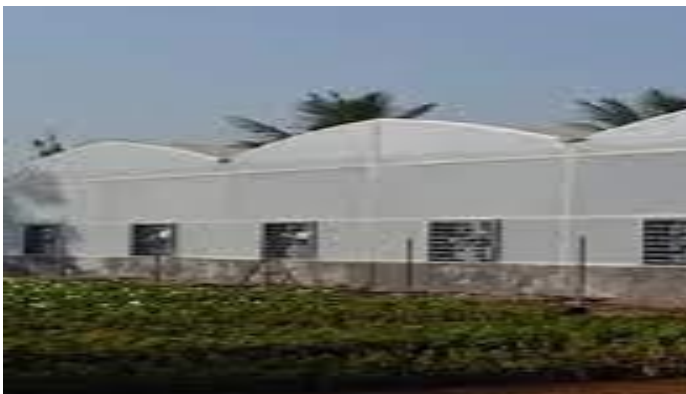
Figure 2: Partially Climate Controlled Polyhouse
