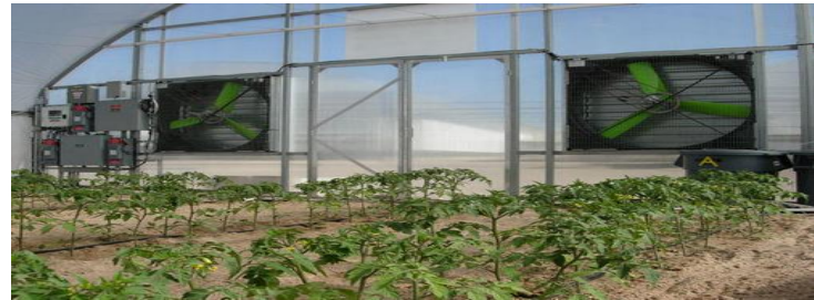
Figure 3: Fully Climate Controlled Polyhouse
