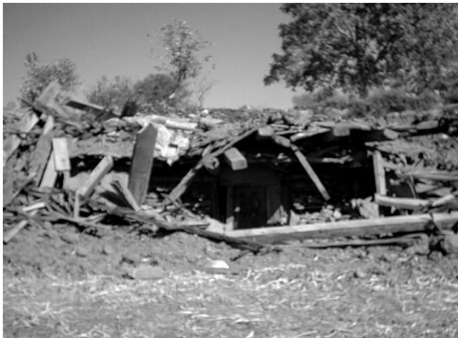
Figure 1: Collapsed house in earthquake with heavy roofing.
