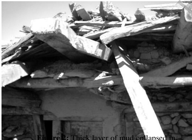
Figure 2: Thick layer of mud collapsed in earthquake
