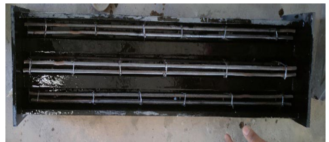
Fig 3.7 Applying Oiling to mould.
