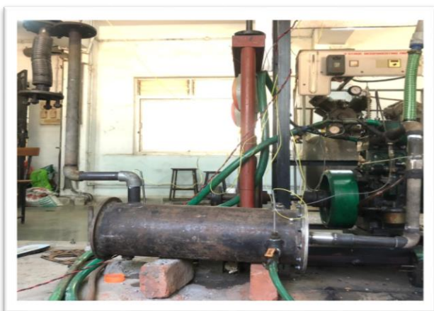
Fig 3 Aqua silencer & heat recovery unit.
