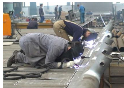
Figure 5. Manual TIG butt welding of pipes on boiler chamber
