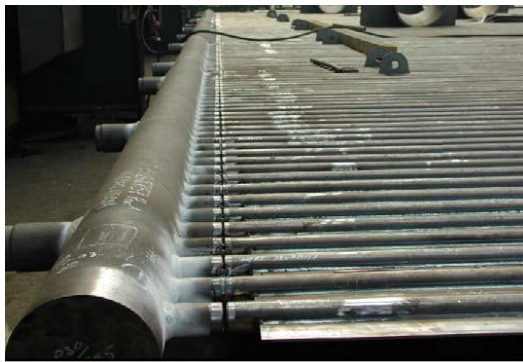
Figure 3. Butt MMA pipe welding of membrane pipe panel-chamber with pipe connectors (nozzles)
