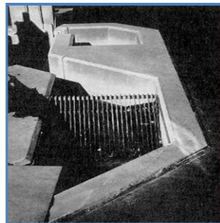
Bar racks and screens remove large solids which could clog pumps and pipes in the wastewater treatment plant. Solids are collected and sent to a landfill.
