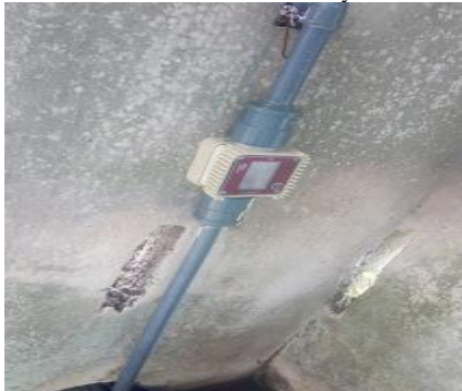
Plate 5: Flow Meter Installation
