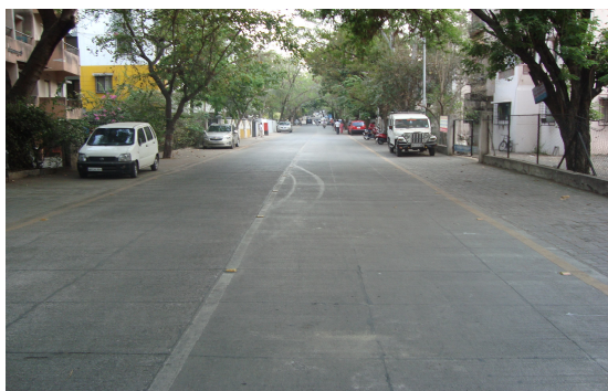
Fig.7: Finished View of UWT Overlay
