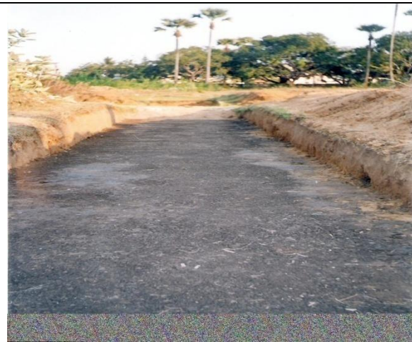
Fig.5 Prepared Expansive Soil Subgrade in the Model Pavement
