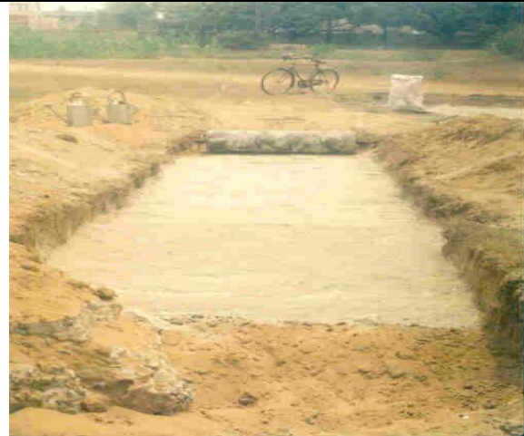
Fig.7 Prepared Flyash Subbase
