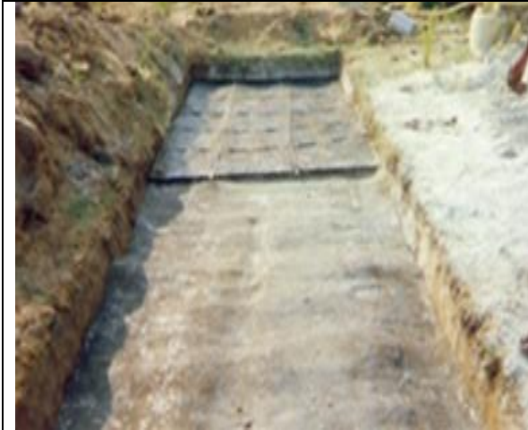
Fig.6 Placing of Reinforcement Material in the Subbase
