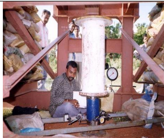
Fig.9 Experimental set-up for conducting Cyclic Load Test
