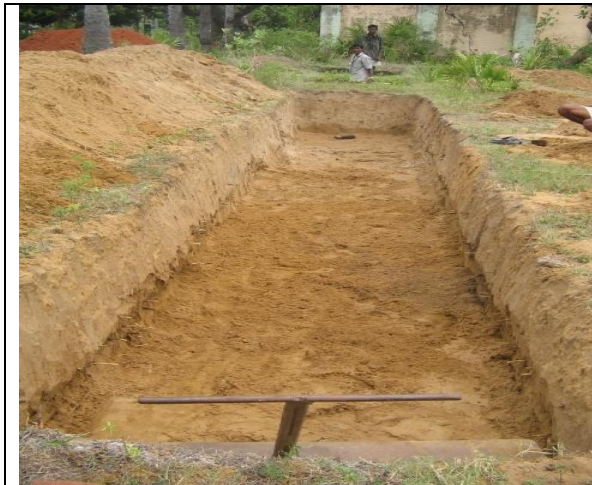
Fig.4 Excavated Model Pavement Stretch
