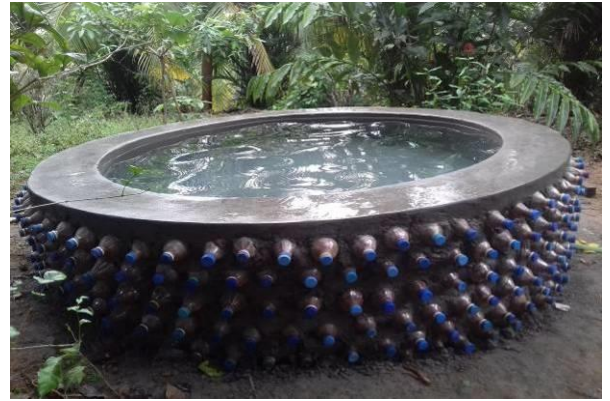
Fig :5 Pet water retaining structure
